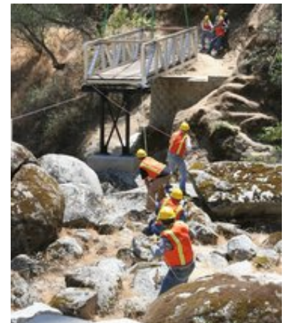
Volunteers maneuver sections of a bridge into place at Big Sandy Creek. "The civilians hadn't done anything like this before. Honestly, we hadn't either," said National Guard Lt. Col. Mark Van Dyke, who piloted the helicopter that hauled the bridge sections. California Department of Parks and Recreation
